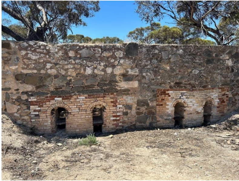
The D-type lime kilns built by George Green in the late nineteenth century.
