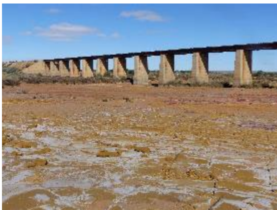
Railway Bridge the Ghan- 1957
