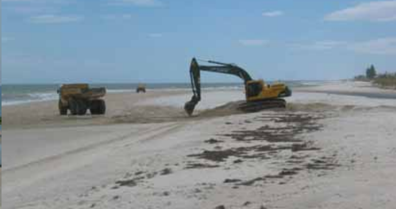
Sand bypassing at the Torrens Outlet (City of Charles Sturt)
