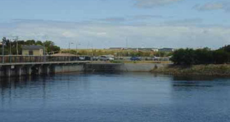
Trash rack over Barcoo Outlet
