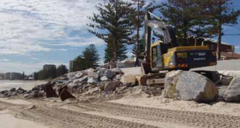
Seawall reconstruction at the Broadway, Glenelg, 2004
