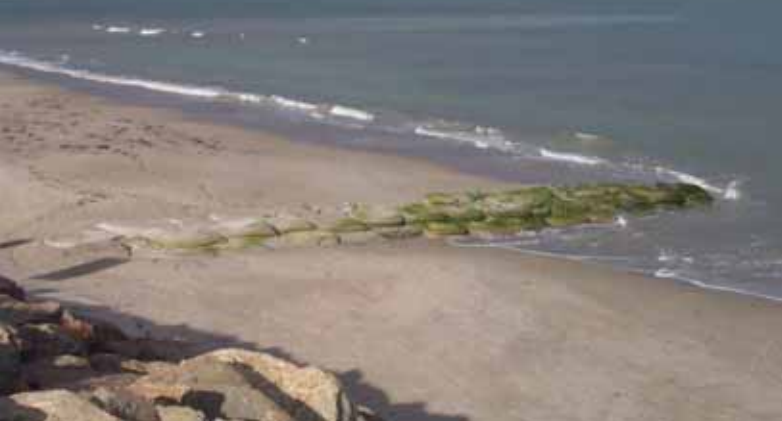
Geotextile groyne at Somerton Park, 2003
