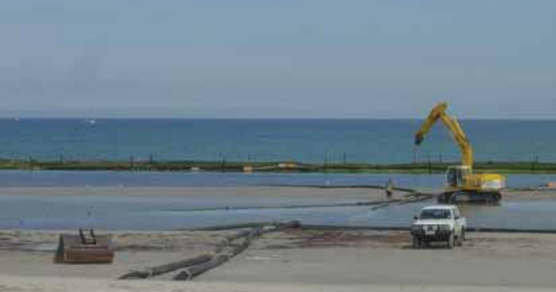
Semaphore South trial breakwater during construction, 2004
