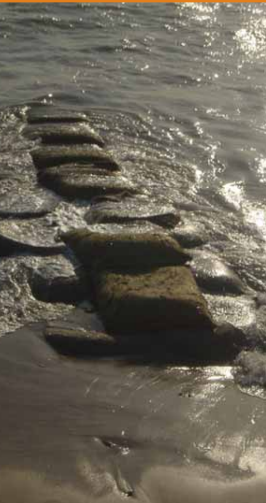
Close-up of a groyne at Somerton Park showing geotextile bag construction
