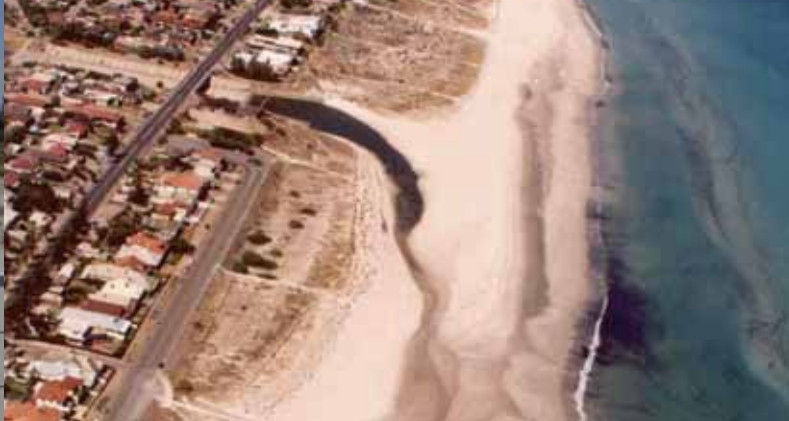
Build-up of sand near the Torrens Outlet
