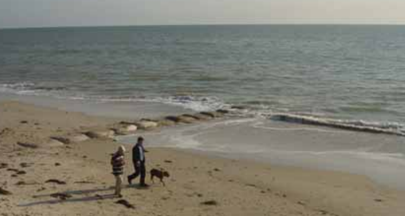
One of the new groynes installed at Somerton Park in 2005
