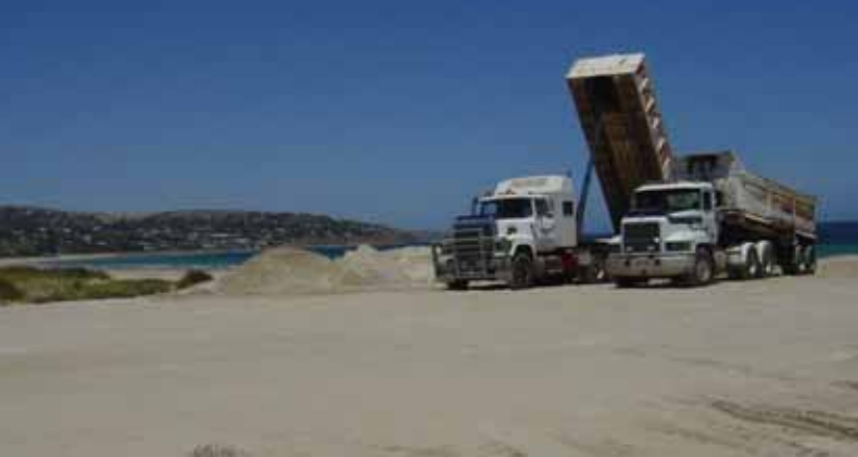
Sand dumping platform at Edwards Street, Brighton
