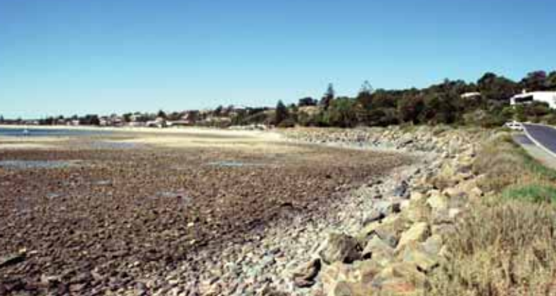
Rip-rap seawall at Seacliff, 2003
