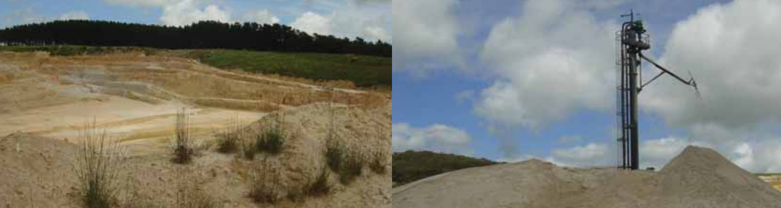
Unimin Sand Plant at Glenshera, Mount Compass
