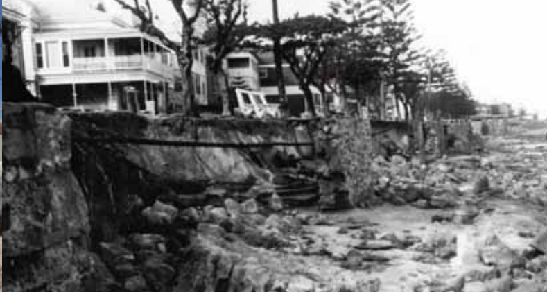
Storm damage at Glenelg, 1960
