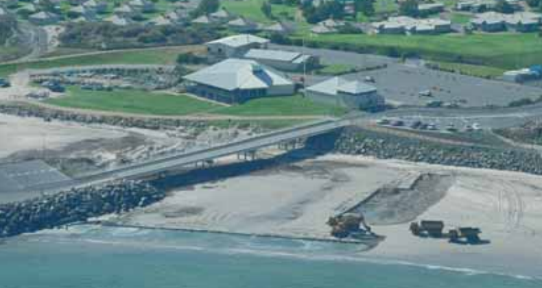
Sand bypassing at Adelaide Shores, West Beach
